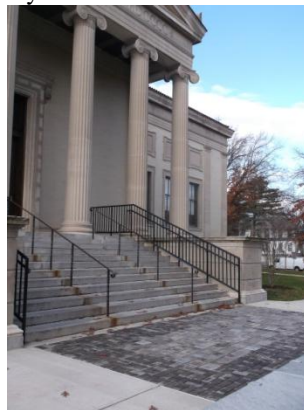
Original Maple St Entrance with brick patio.
